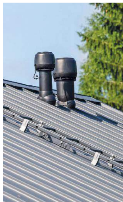
Wentylatory na dachu stromym
